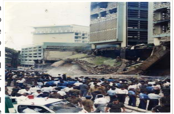
LTTE attacked central bank of Sri Lanka in 1996 with an explosive laden lorry. Over 100 people were killed and 1200 others suffered injuries
